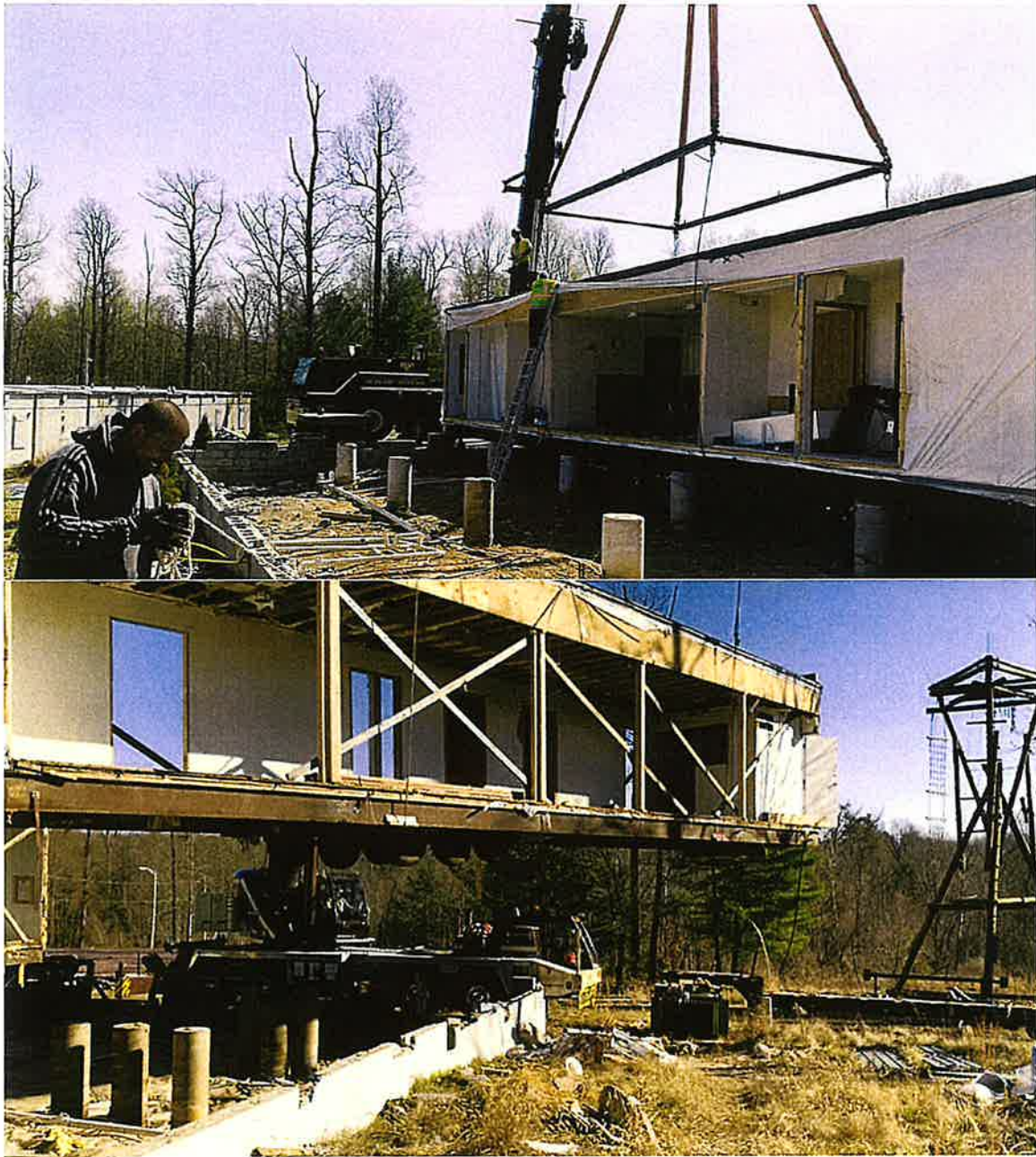
Its HVAC Equipment and flex duct was removed by Fowler HVAC
